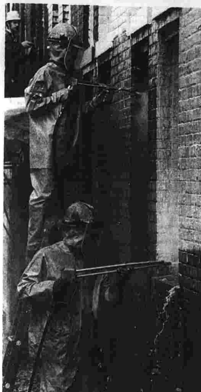
Store restoration begins
